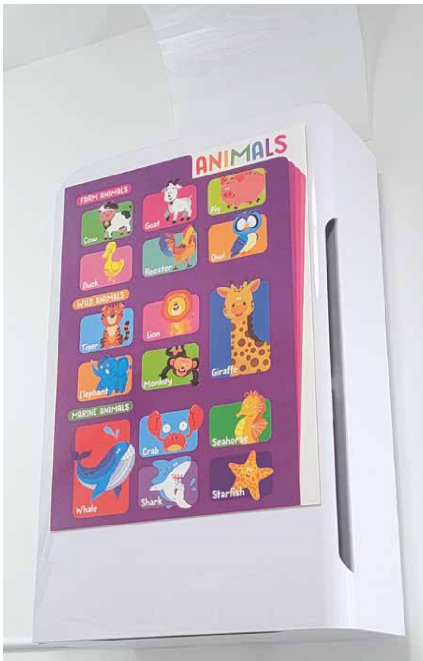
A high wall-mounted HEPA/UV-C Air Purifier, one of three in a smart classroom system.
